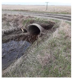
This picture is an example of a culvert that is too short for its location, causing in-channel erosion and destabilization of the road approach.
