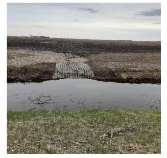
In partnership with Traverse SWCD, lined concrete mats are used to stabilize field outlets.
